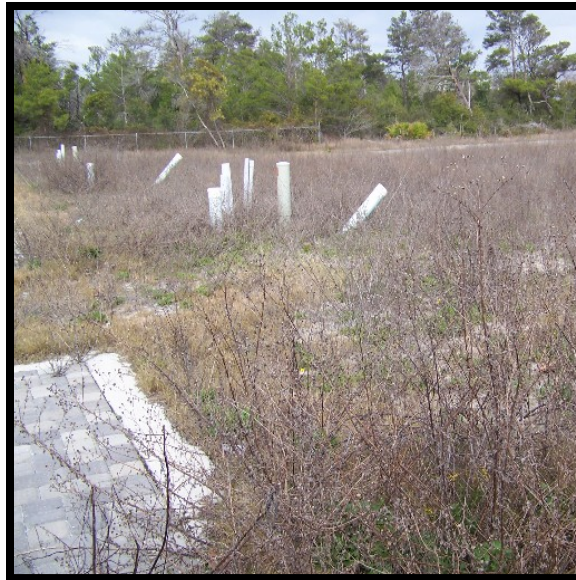
Was this subdivision completed properly?
